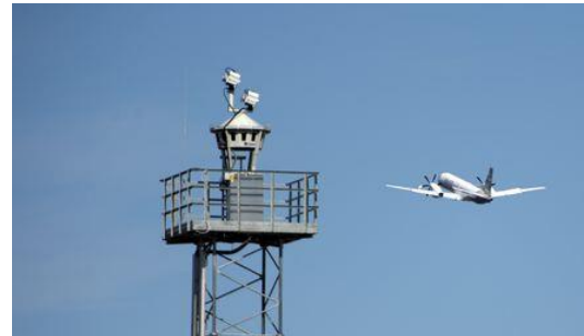
World's first remotely controlled ATCT at Ornskoldsvik Airport, Sweden. Source: Stefan Kalm at Saab AB.
