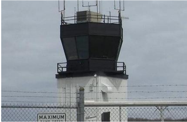
Ithaca-Tompkins Airport (ITH) Control Tower, Ithaca, NY Source: www.flickr.com
